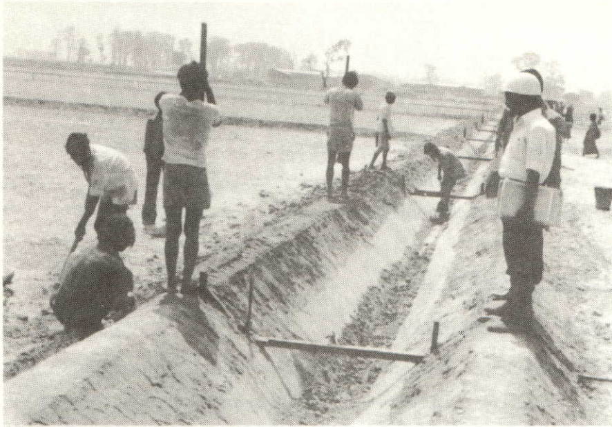
ASS Canal Excavation
