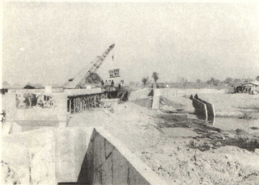
Trunk Road No. 3 Bridge Concrete Placing
