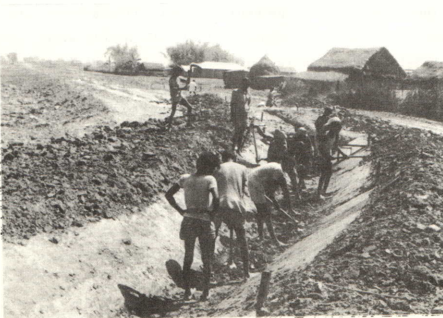
SIC Excavation Feb. '78
