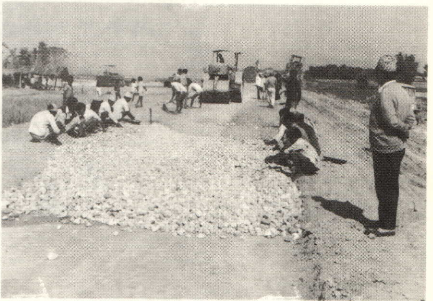
Trunk Road Gravel Pavement
