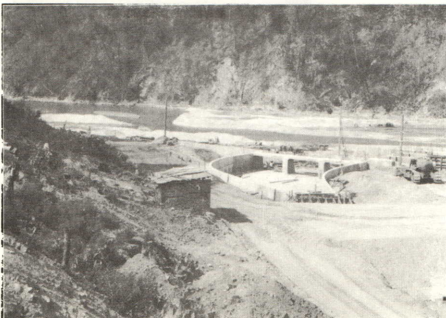
Diversion Weir Intake
