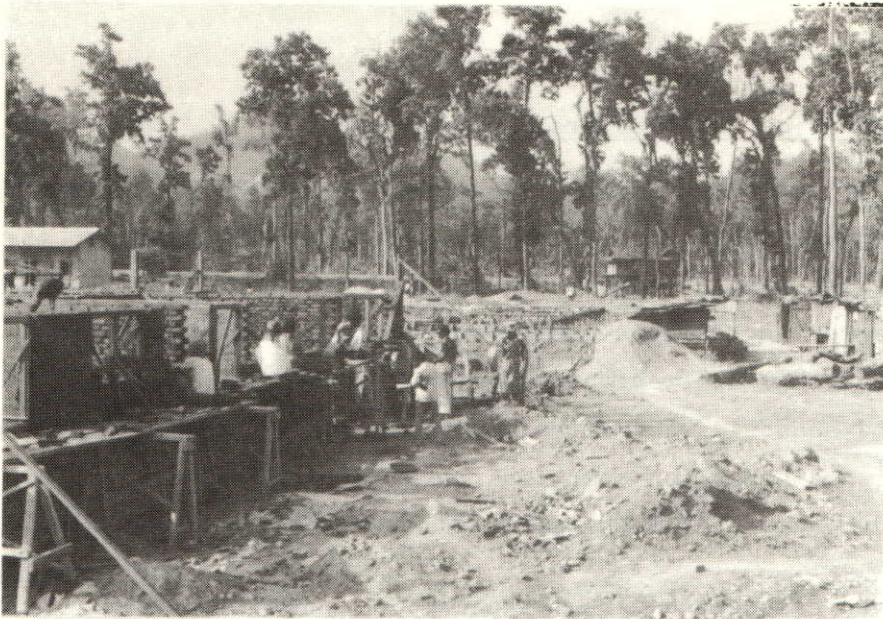
EOQ Building Construction Apr. '75
