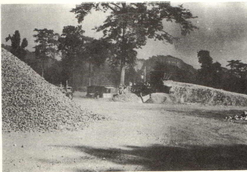
Crushing Plant at Dudhe
