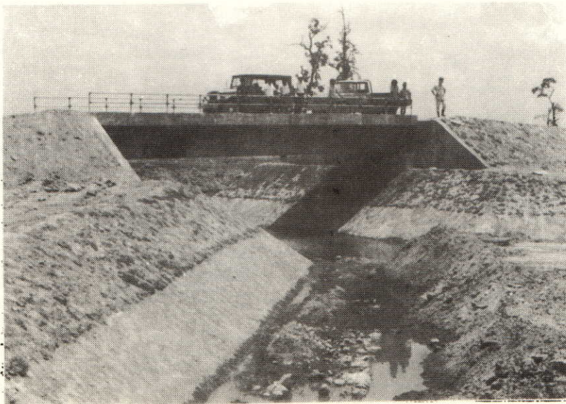
Trunk Road No. 2 Bridge Completed
