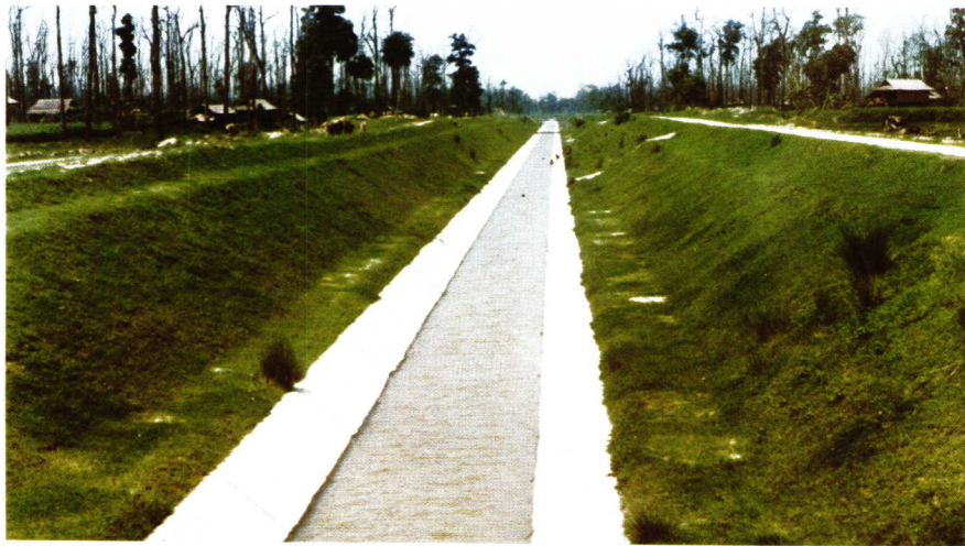
Main Irrigation Canal
