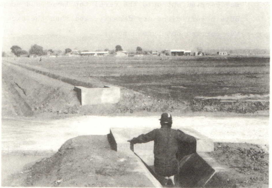
ASS Canal Earthworks & Land Readjustment
